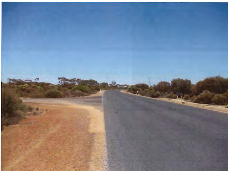
Photograph 6 View West along Brookton Hwy , showing ENTRY/EXIT driveway on left
